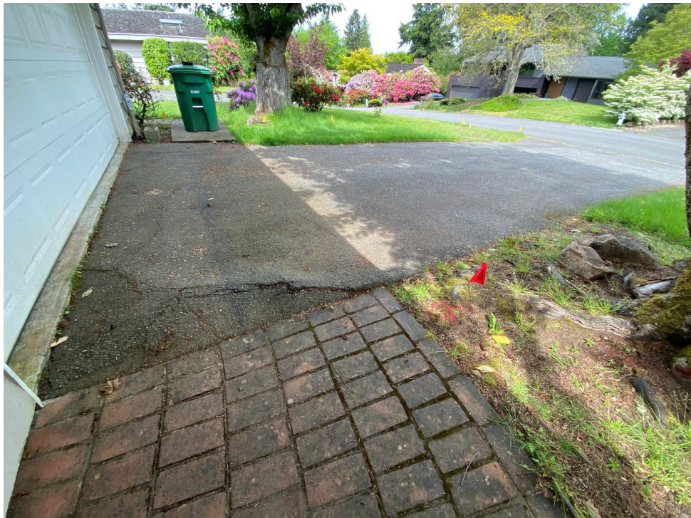
Photo # 3: Looking at the base of tree # 244 on the far side of the driveway and the damage being done to the driveway and sidewalks.
